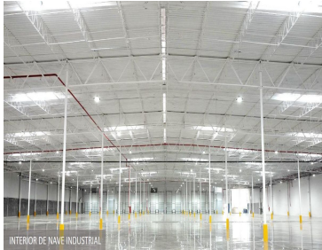
INTERIOR DE NAVE INDUSTRIAL
