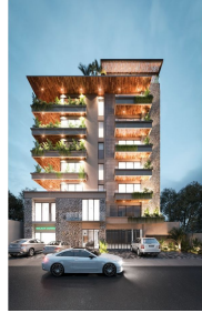
Fachada de noche Facade by night
