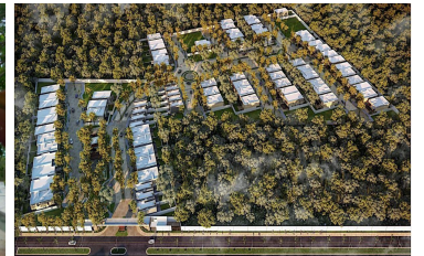
Vista Aérea del residencial Gated community aerial view
