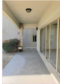
Terraza techada en planta baja Roofted terrace in ground floor
