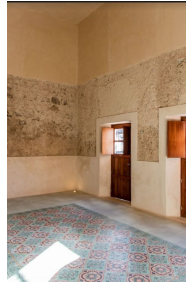
Techo alto High ceiling
